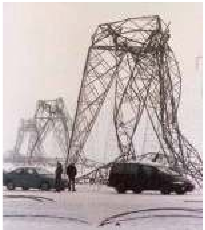
Figure 1 Dramatic evidence of the power of ice on the power industry. One hundred foot tall towers carrying power lines are seen here bent like blades of grass in the aftermath of the 1998 ice storm that hit southeastern Canada and the Northeastern US.
